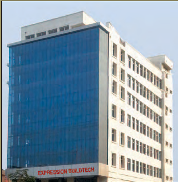
Completed project at Kankarbagh Road, Patna
